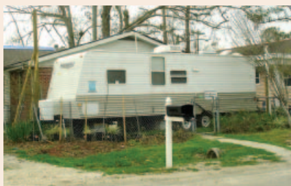
A trailer in front of a storm-damaged home in Louisiana.
